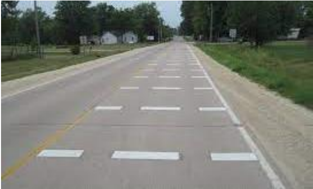
Figure 36: Transverse Markings with Speed Bars
