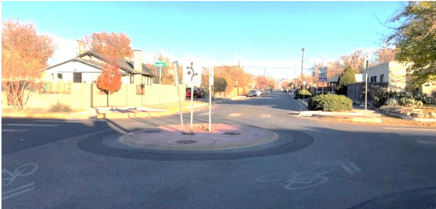
Figure 34: Mini-Roundabout Example, Silver Ave Near the University of New Mexico
