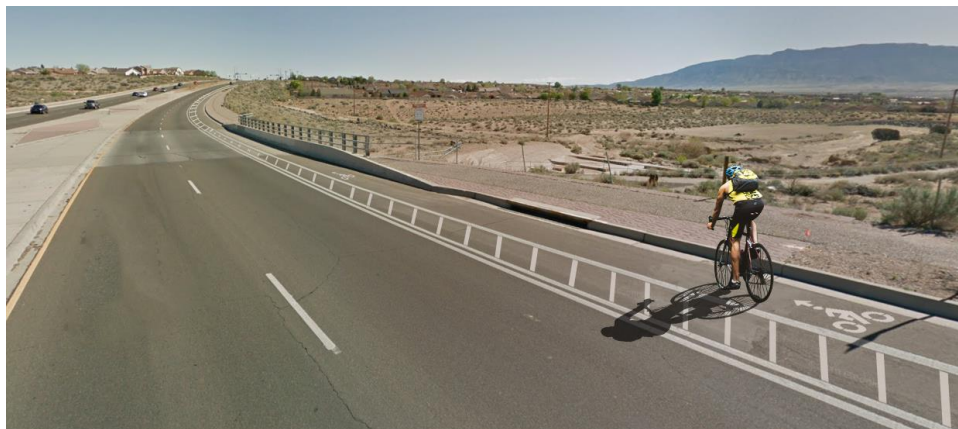
Figure 33: Buffered Bike Lane Rendering, Unser Blvd
