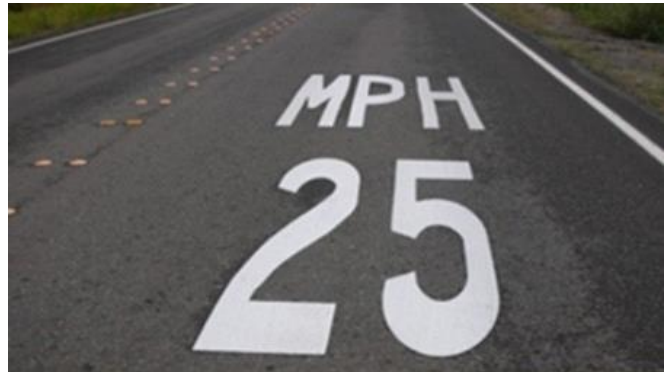
Figure 37: Enhanced Pavement Markings
